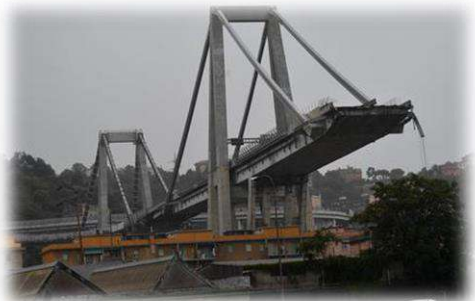
Morandi bridge collapse (Italy)
