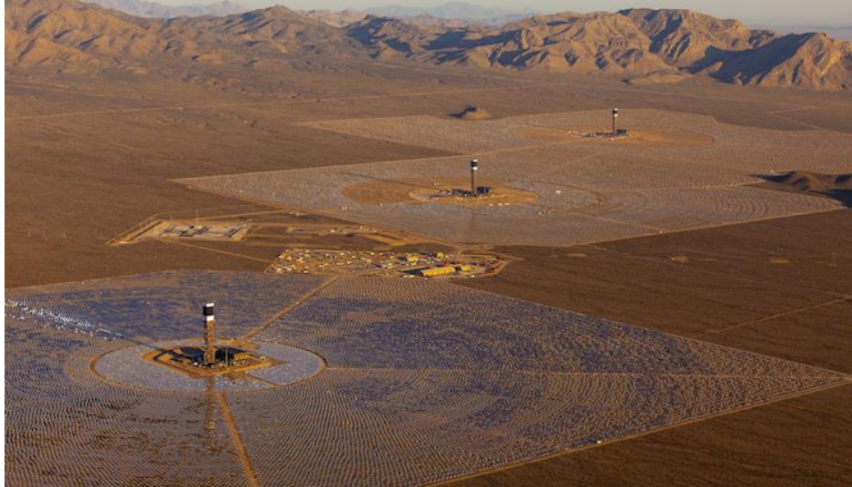
Ivanpah Solar Electric Generating System
